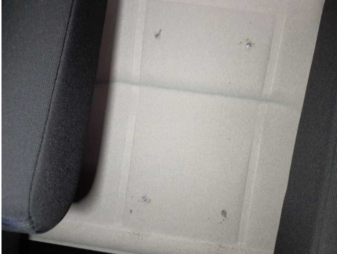
Damage 7: Body: Partition wall - Holes - Replace
