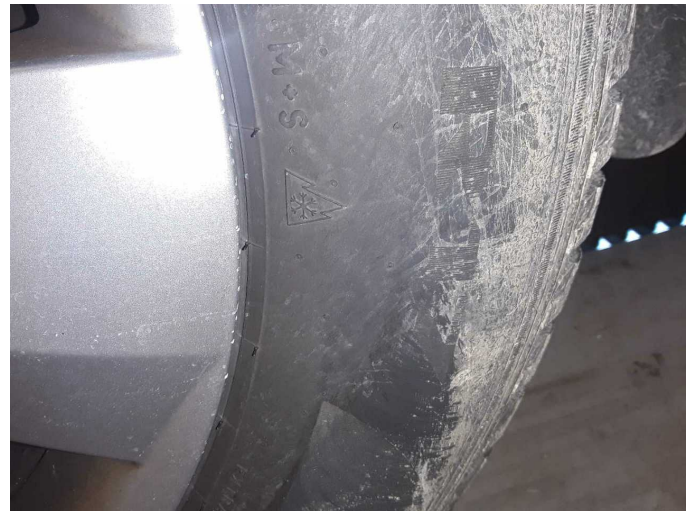
Damage 4: Wheel / tyres: Tyre - front (2x) - Does not meet the leasing specifications - Replace
