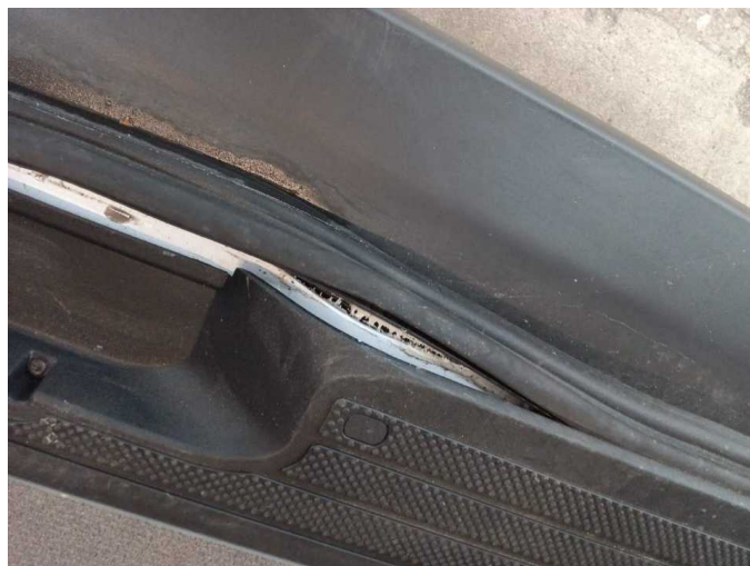
Wear and tear 4: Boot lid / rear door: Seal - Malposition - Replace
