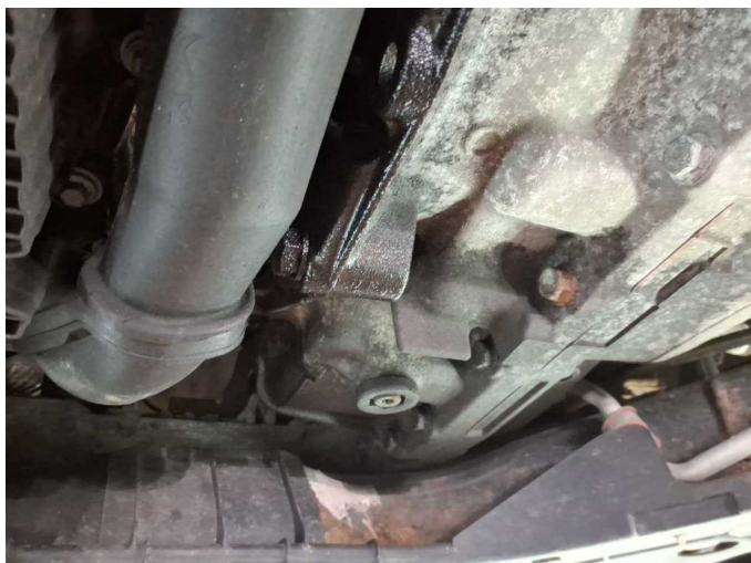
Damage 1: Gearbox: Gearbox - Leaking - Perform diagnosis
