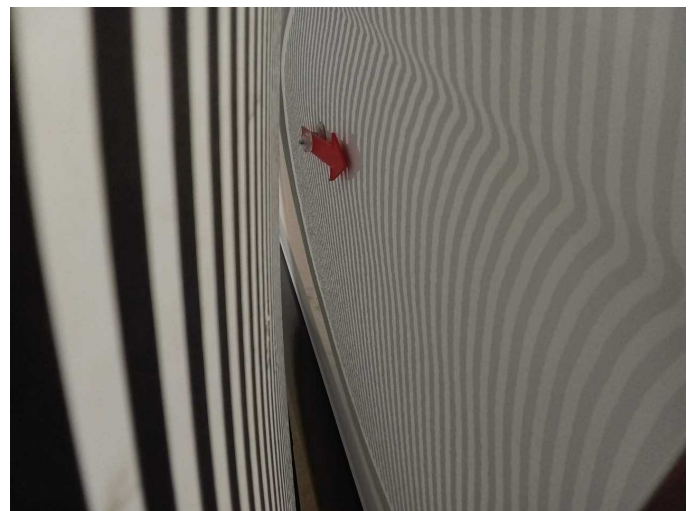
Wear and tear 6: Sliding door, right: Sliding door - dent(s) - No deduction
