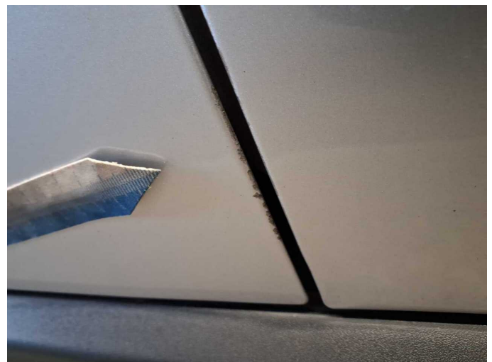
Damage 9: Door - front left side: Door (Verformt innen) - Dent / paintcoat damage - Repair and paint
