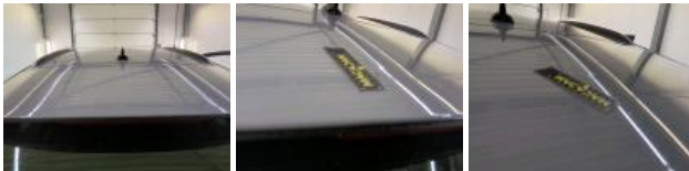
Roof, Dent(s), Repair and paint (complete)
