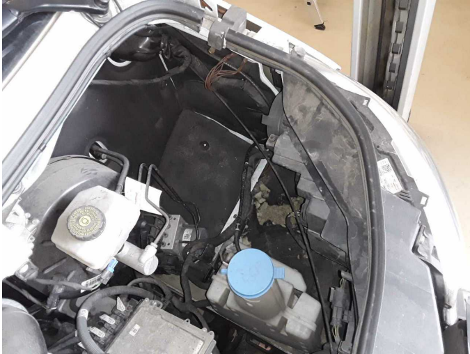
Damage 1: Cab: Insulation lining (Im Motorraum) - Broken / torn - Replace
