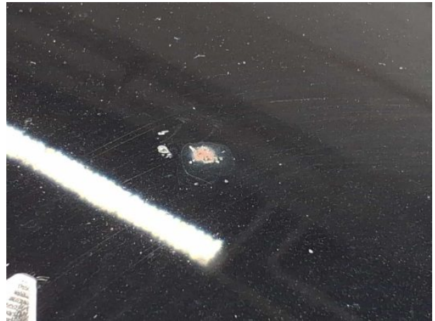
Damage #13: Roof: Roof - Corrosion - Repair and paint
