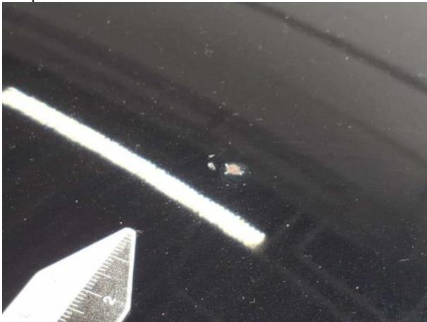
Damage #13: Roof: Roof - Corrosion - Repair and paint
