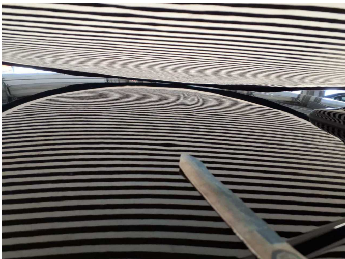
Damage 1: Roof: Roof - dent(s) - Smooth repair work
