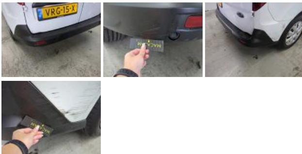
Parking sensor R, Deformed / Strained, Replace
