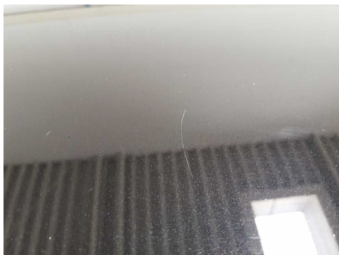
Damage 17: Roof: Roof - Dent / paintcoat damage - Repair and paint
