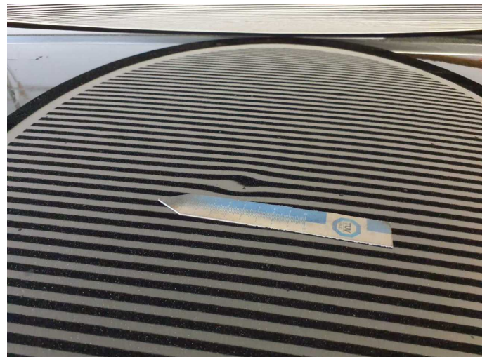
Damage 4: Roof: Roof - Damage by hail - Smooth repair work
