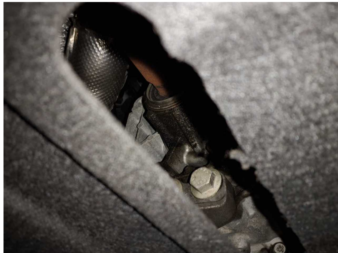
Damage 2: Gearbox: Gearbox - Leaking - Perform diagnosis
