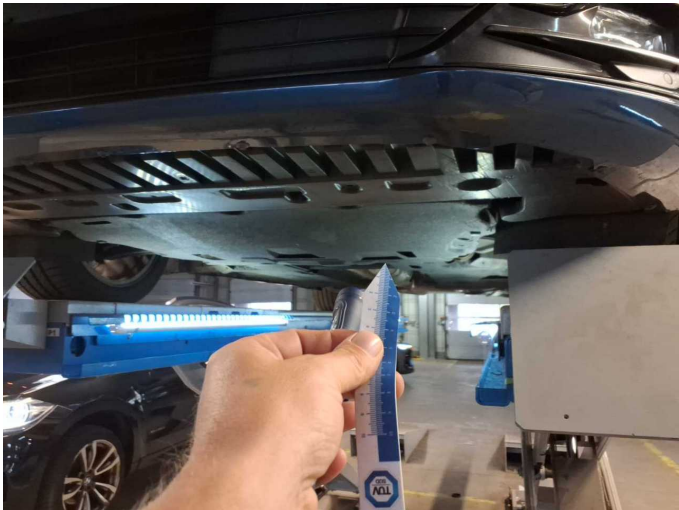
Damage 2: Gearbox: Gearbox - Leaking - Perform diagnosis
