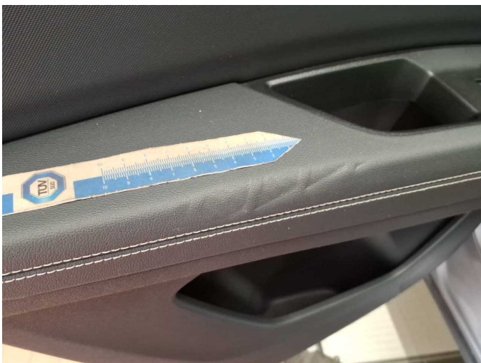
Damage 4: Trim / covers: Door trim - rear left side - Deformed - Loss in value
