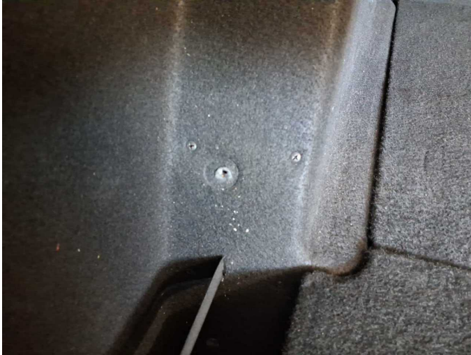
Damage 9: Trim / covers: Cargo area - lining -left side (Fehlbohrungen) - Differs from the original configuration - Replace
