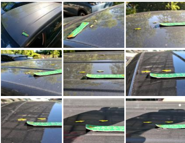
Roof, Hail damage, Repair and paint (complete)
