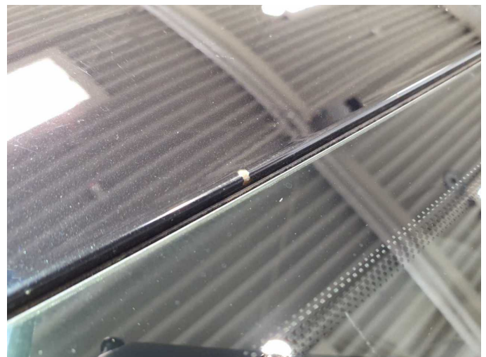
Damage 15: Roof: Roof - Corrosion - Paint
