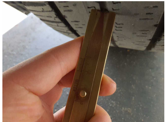
Damage 7: Wheel / tyres: Tyre - right (Keine Winterreifeneigenschaften) - Does not meet the leasing specifications - Replace
