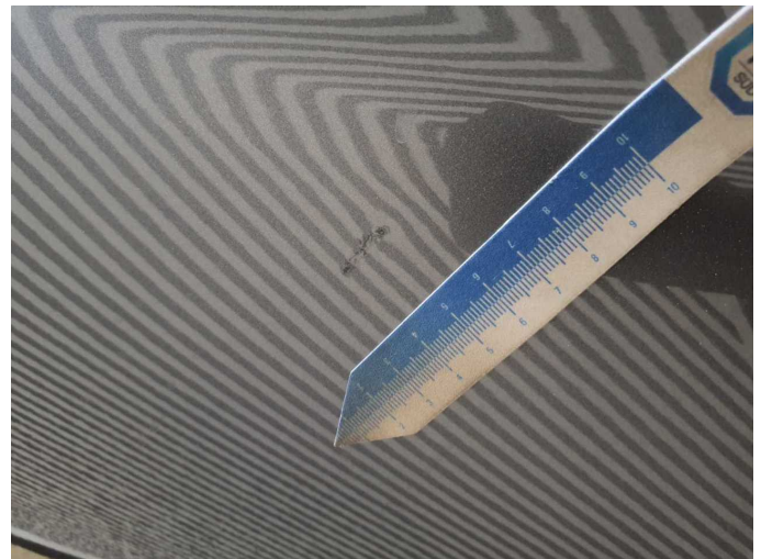
Damage 5: Door - front right side: Door - Dent / paintcoat damage - Repair and paint
