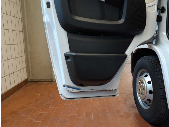
Damage 7: Door - front left side: Door (Unten / innen) - Corrosion - Loss in value
