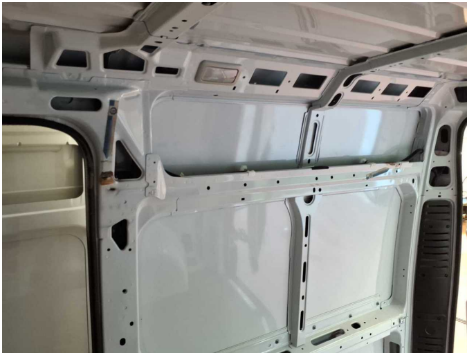
Damage 10: Side panel - rear right side: Side panel (Innen) - Corrosion - Smart repair
