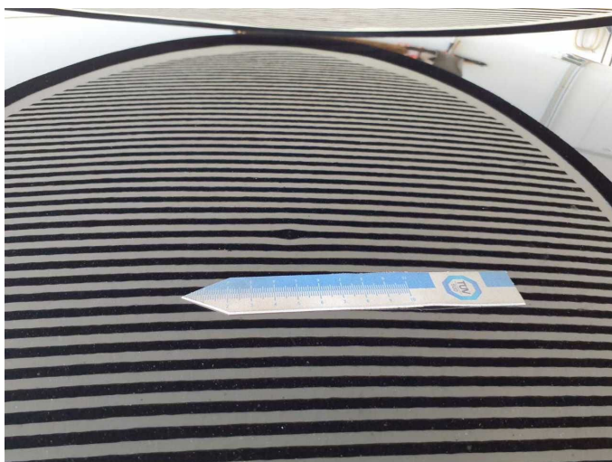
Damage 7: Roof: Roof - dent(s) - Smooth repair work
