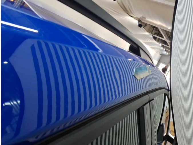
Damage 1: Roof: Roof rail - right side - dent(s) - Smart repair
