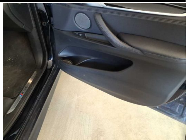
Damage #9: Trim / covers: Door trim - front right side - Damaged - Loss in value
