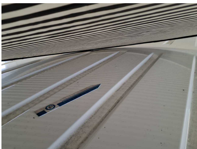
Damage 4: Roof: Roof - dent(s) - Smooth repair work
