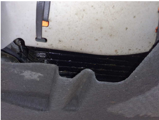
Damage 2: Gearbox: Gearbox (Ölverlust) - Leaking - Perform diagnosis
