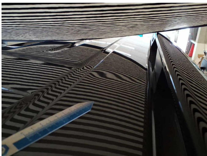
Damage 6: Roof: Roof - dent(s) - Smooth repair work
