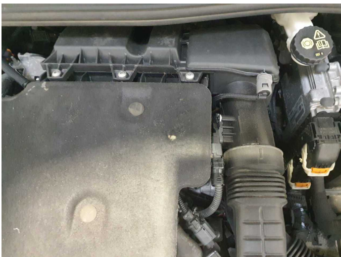
Damage 5: Bonnet: Insulation lining - Broken / torn - Replace
