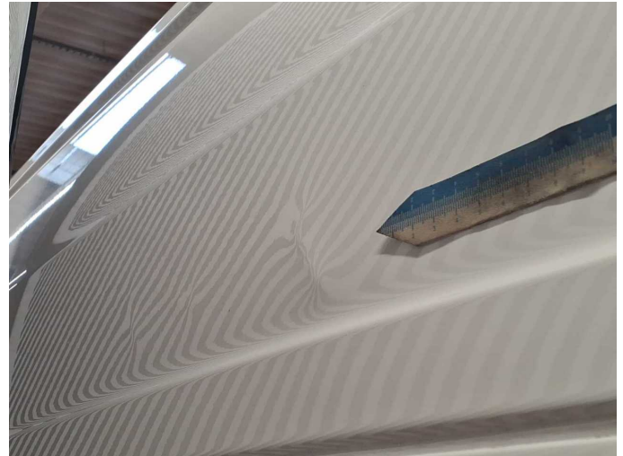
Damage 5: Side panel - rear right side: Side panel - dent(s) - Repair and paint
