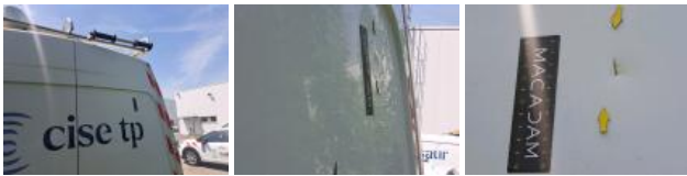
Other exterior parts, Missing, Replace
