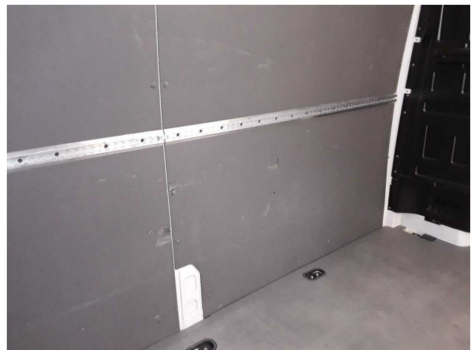
Damage 3: Side panel - rear left side: Interior trim - Broken / torn - Replace
