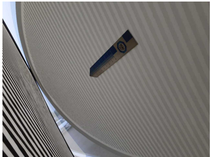
Wear and tear 7: Side panel - rear right side: Side panel - dent(s) - Smooth repair work
