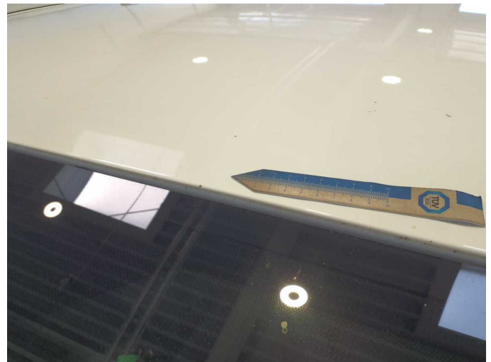
Damage 2: Roof: Roof - Stone chips - Smart repair
