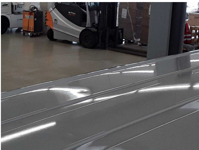
Damage 8: Roof: Roof - dent(s) - Smart repair
