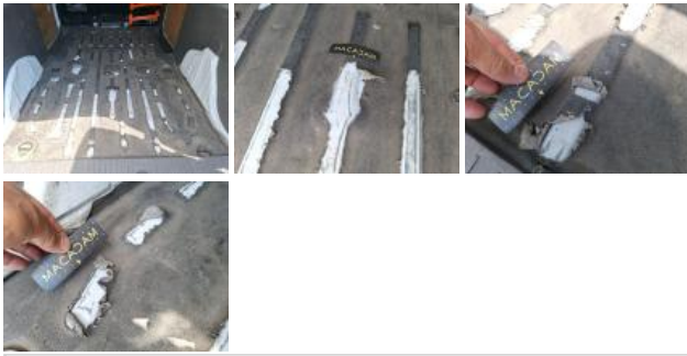
Reflector, Broken, Replace
