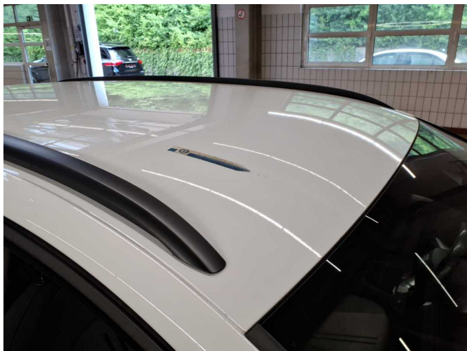
Damage 13: Roof: Roof - Corrosion - Paint
