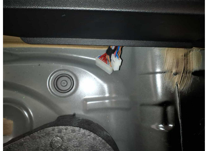
Damage 5: Electrical system: Cable strand (Kabelführung von Frontbereich in Laderaum) - Differs from the original configuration - Remove
