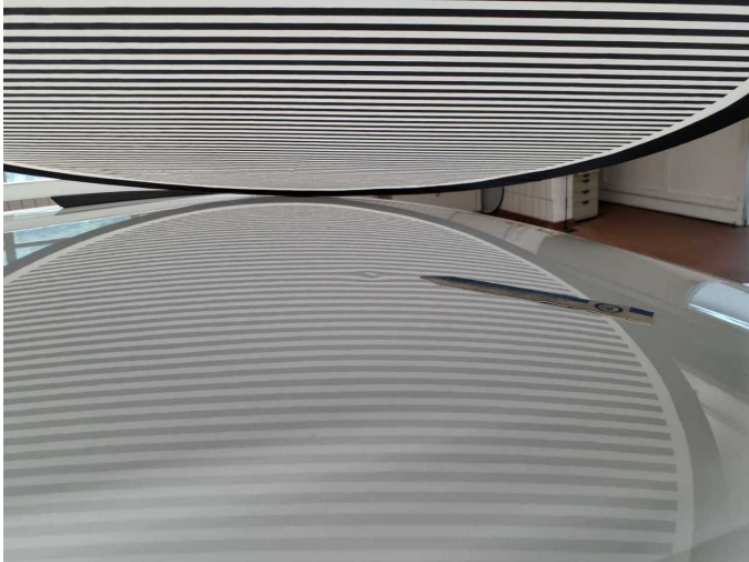
Damage 2: Roof: Roof - dent(s) - Smooth repair work
