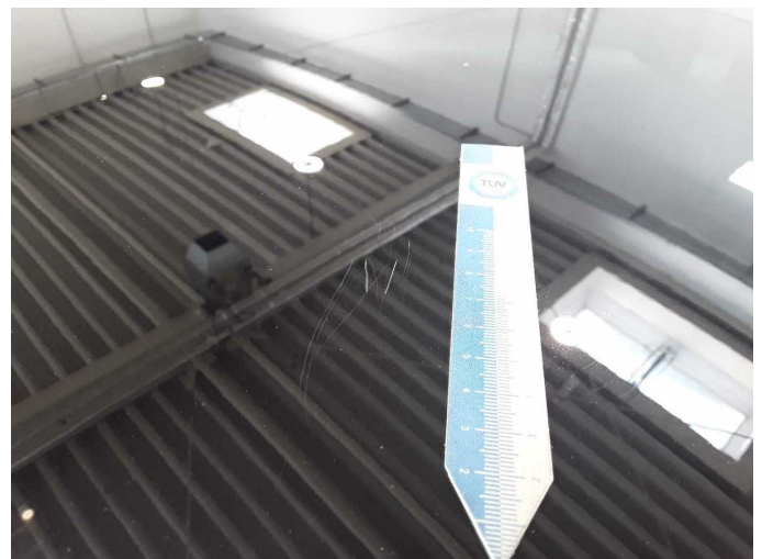
Damage 4: Roof: Roof - Scratch(es) - Paint
