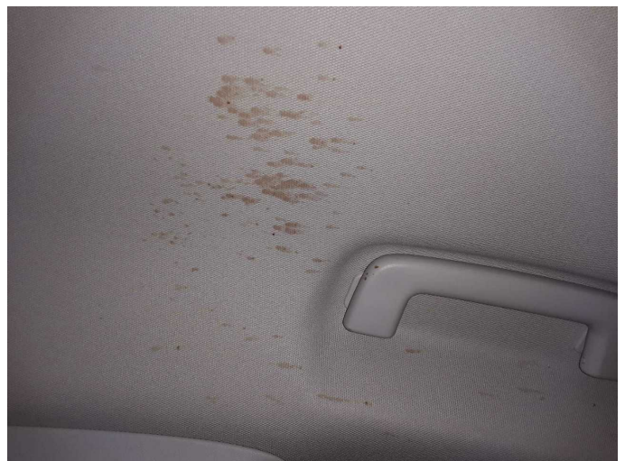
Damage 1: Trim / covers: Roof lining - Soiled - Clean
