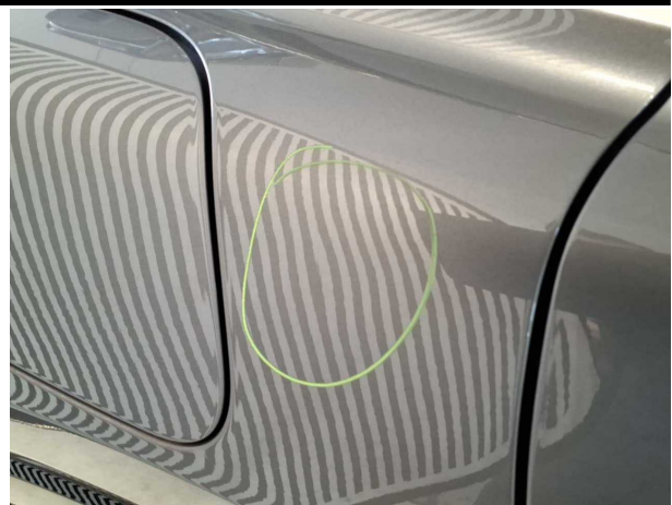
Damage #10: Side panel - rear right side: Side panel - dent(s) - Smooth repair work
