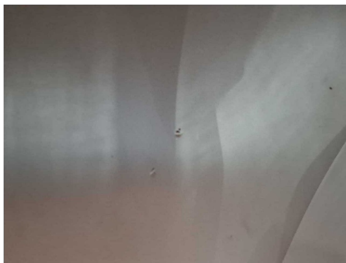
Damage 19: Trim / covers: Roof lining - Scratched - Loss in value
