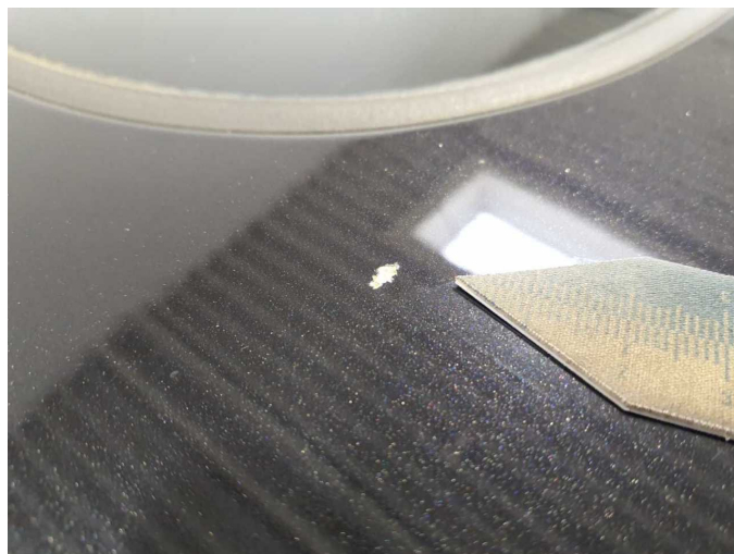
Damage 12: Roof: Roof - Corrosion - Paint
