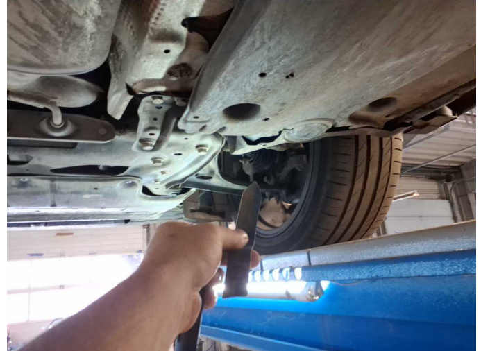
Damage 10: Drive train: Sleeve prop shaft - front right side (Fett tritt aus) - Loose - Replace
