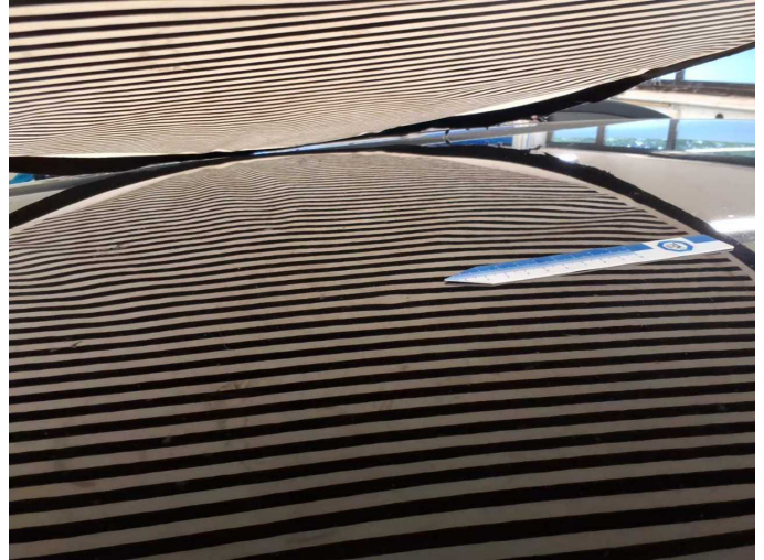
Damage 6: Roof: Roof - dent(s) - Smooth repair work
