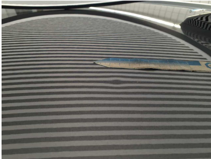
Damage 5: Roof: Roof - dent(s) - Smooth repair work
