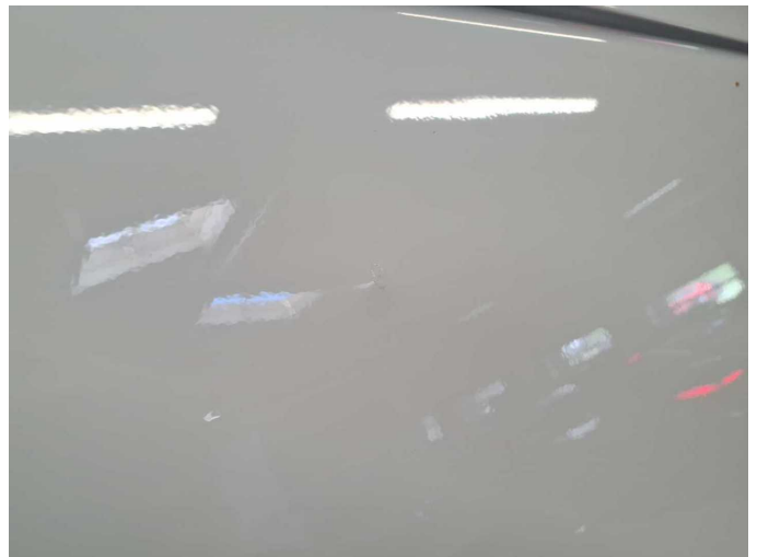
Damage 12: Side panel - rear left side: Side panel - Deformed - Repair and paint
