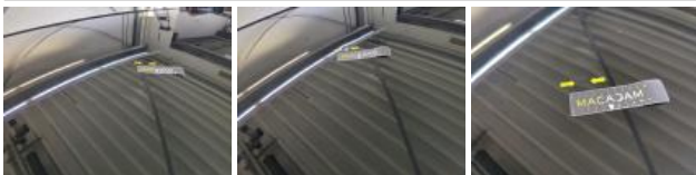
Roof, Dent(s), Repair and paint (complete)
