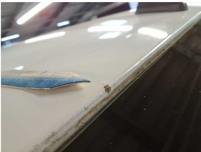
Damage 10: Roof: Roof (Korrosion) - Stone chips - Paint
