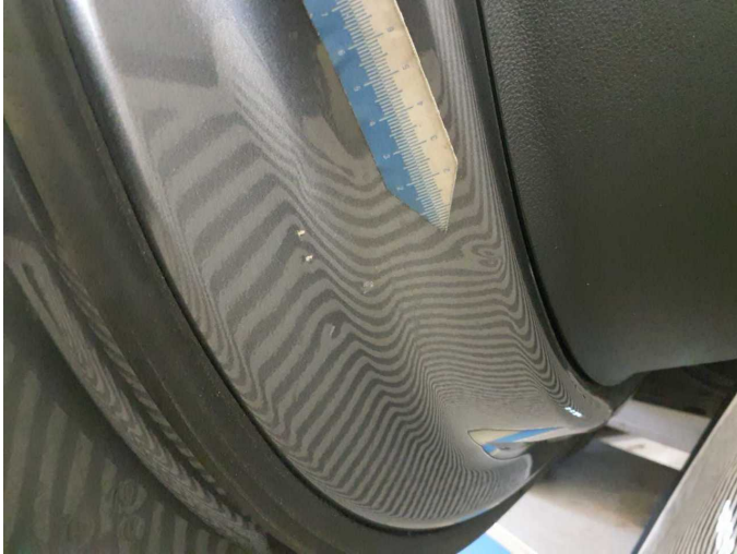
Damage 6: Door - front left side: Door (Innen) - Dent / paintcoat damage - Smart repair
